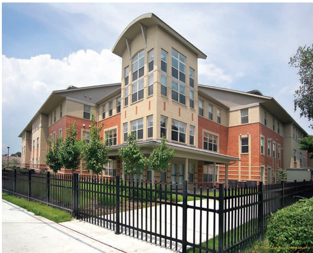
FIGURE 18. Union Court Elderly Apartments
