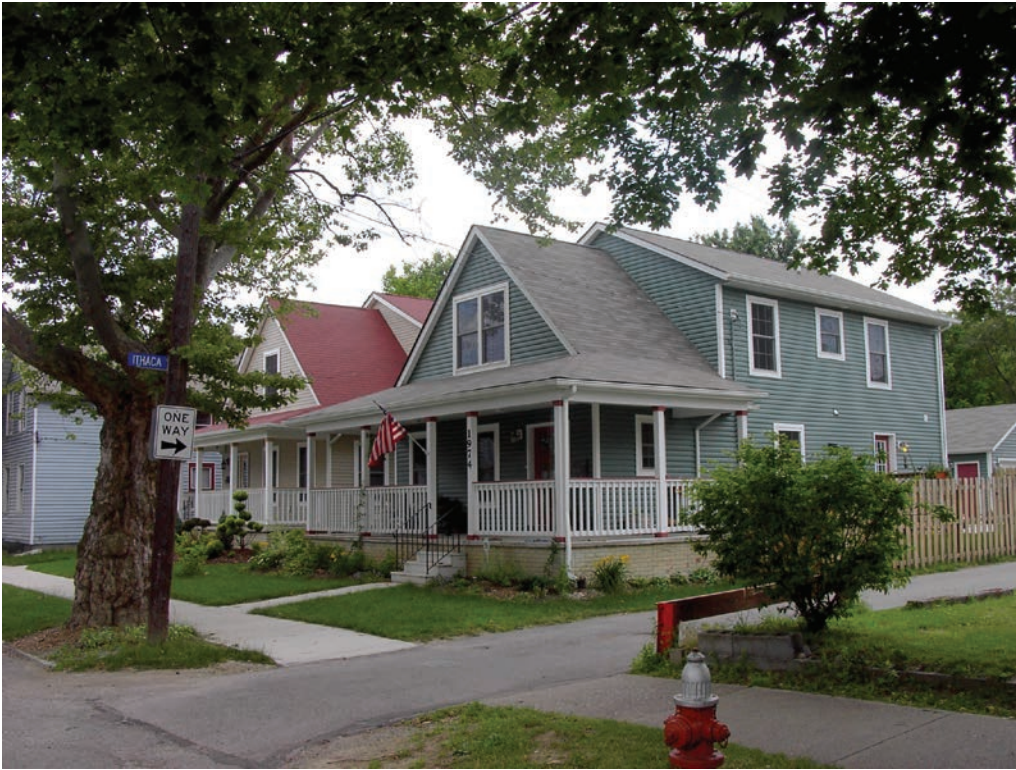
FIGURE 22. Detroit Shoreway EcoVillage includes green rehabilitation of historic homes in the neighborhood.
