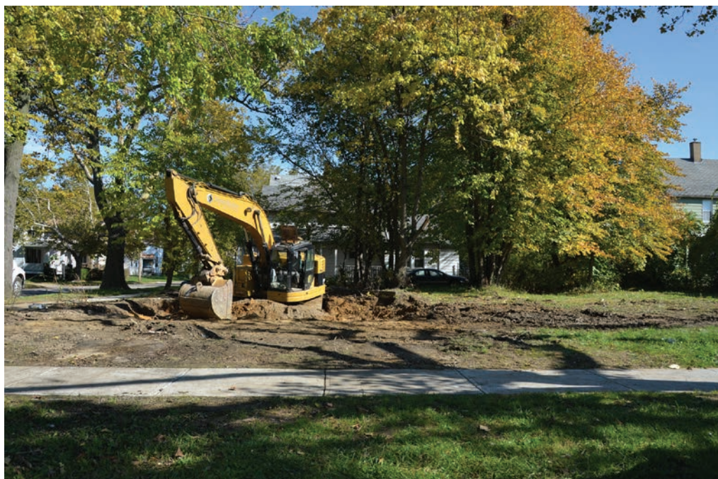
Figure 11. Policies and programs to secure and demolish abandoned structures must be among the city and county strategies for addressing vacancy, especially in cities where vacancy has persisted for decades.
